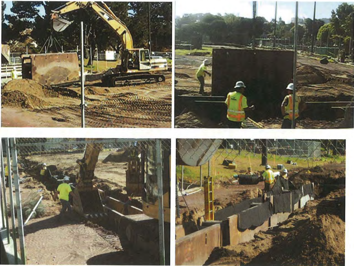
Kimball Field (SF), synthetic field "pour forms" placement
